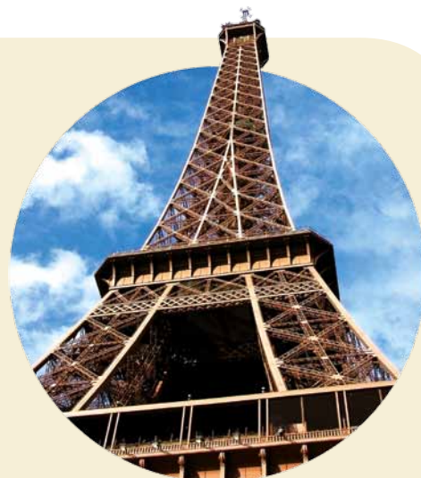
Figure 4 The Eiffel Tower in Paris is made from steel, an alloy of iron.
